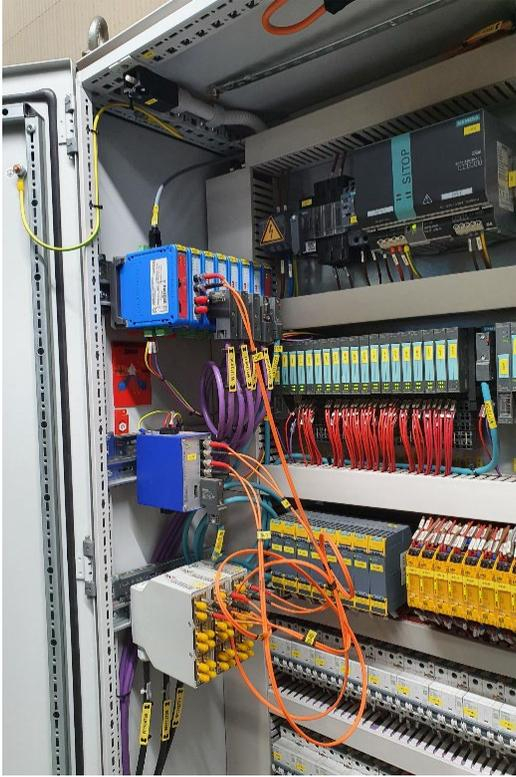
Figure 142: PROFIBUS devices (ComBricks) inside the cabinet
