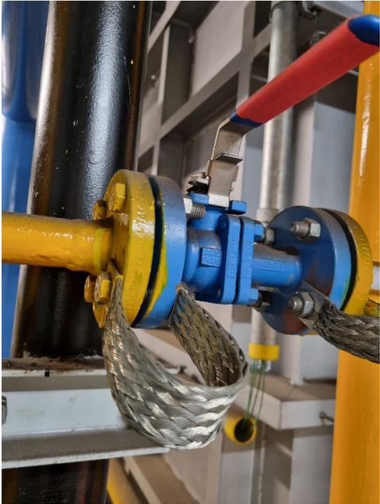
Figure 137: Litz wires on the gas installation (2)
