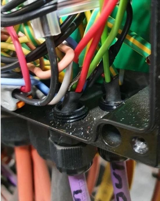
Figure 145: PROFIBUS cables entering the Dungs cabinet
