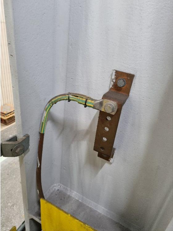
Figure 138: PE connection to the building's earthing
