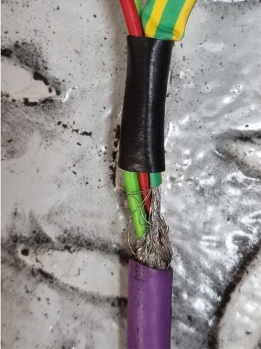
Figure 146: Detail of the PROFIBUS cable (1)
