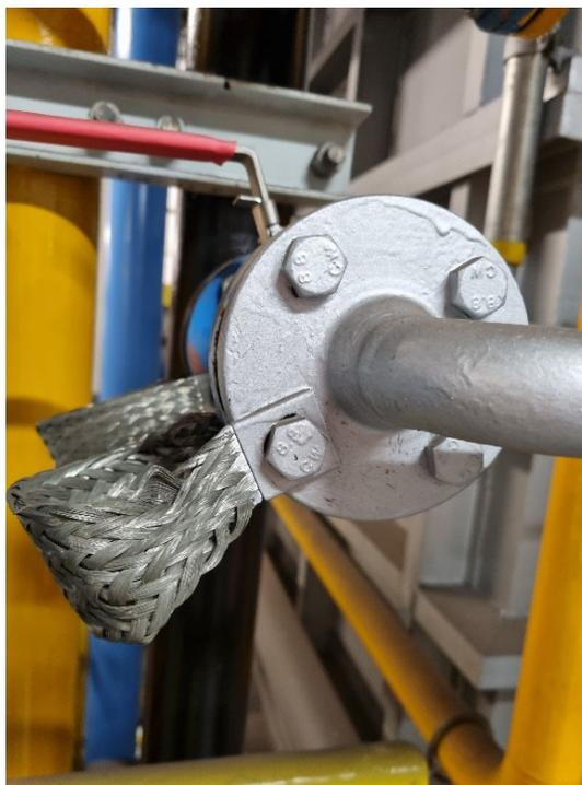
*Figure 136: Litz wires on the gas installation (1)*
